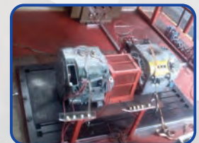
0 - 6600V AC & DC High Voltage Test Bench
